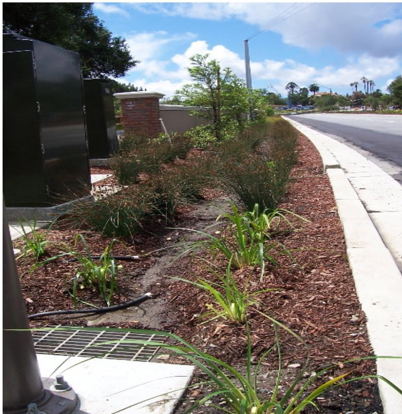
**Figure 16.** Vegetated swale along Sand Hill Road. Road runoff is diverted to the swale through curb cuts (see Figure 17). The swale drains to a catch basin before entering San Francisquito Creek.
