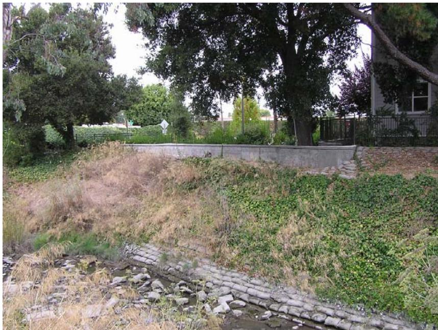
**Figure 28.** Woodland Creek Apartments. Showing location of proposed flow-through path designed to accommodate increased runoff from the project. The wall in the center of the photograph will prevent a flow-through path from functioning during high flows,
