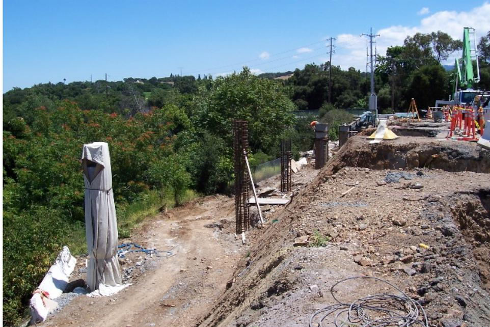
**Figure 10.** Bridge expansion project on San Francisquito Creek, Junipero Serra Boulevard. The project entirely avoided the riparian zone. Extensive erosion control measures were applied at the periphery of the excavated area.
