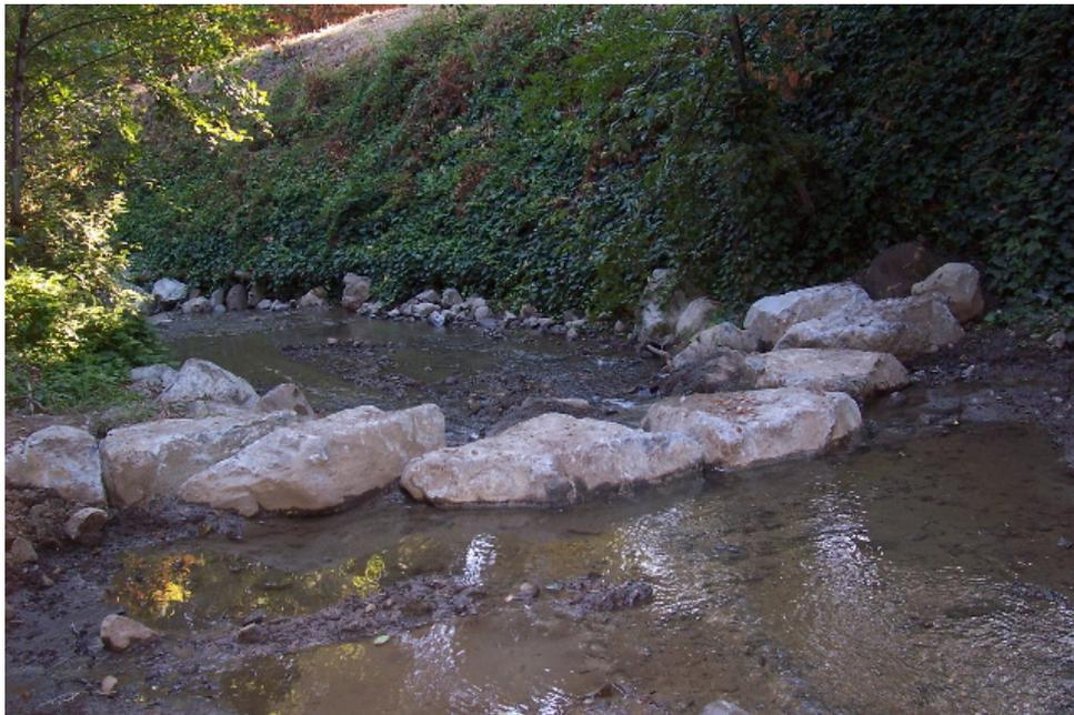
**Figure 5.** One of five weirs installed to reduce bank erosion and incision on Saratoga Creek. This type of treatment is being applied by SCVWD as an alternative to typical bank stabilization approaches.
