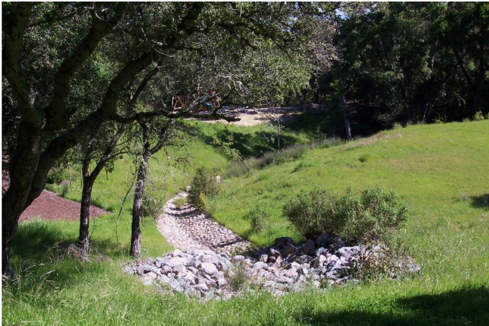
**Figure 22.** Rock-lined drainage swale, Blue Oaks subdivision.
