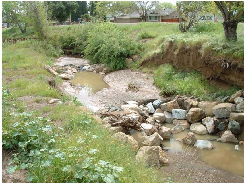
**Figure 6.** Cross vane weirs promoting deposition and channel narrowing, Thompson Creek.
