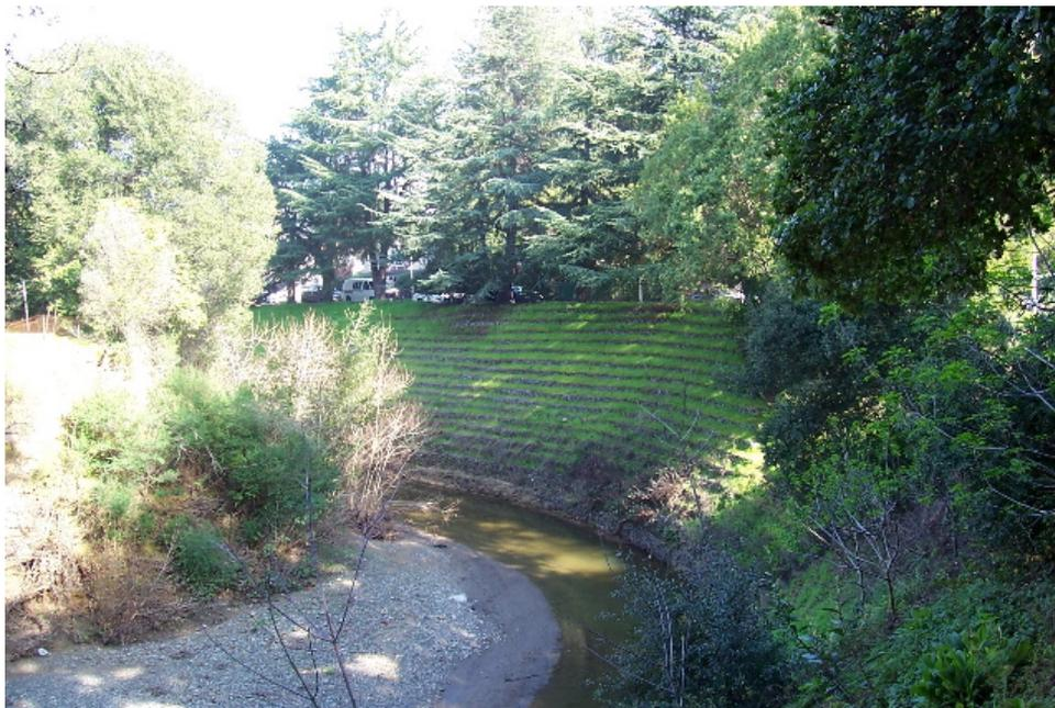
**Figure 2.** Gabion bank protection on San Francisquito Creek, Palo Alto. Bank protection is variable and interspersed with natural channel throughout the watershed on the main stem and tributaries.
