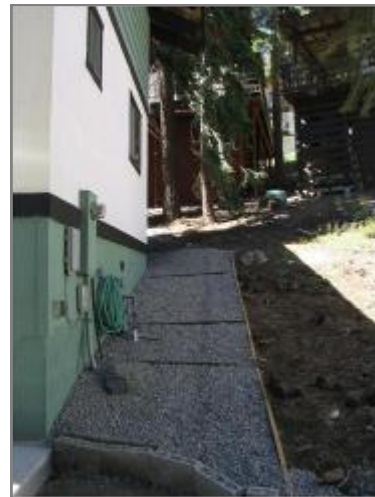
Sample eave line dissipation and infiltration options
